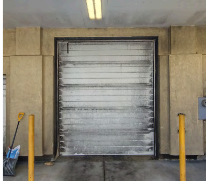
Impact damage, cracks, stained lamina.
