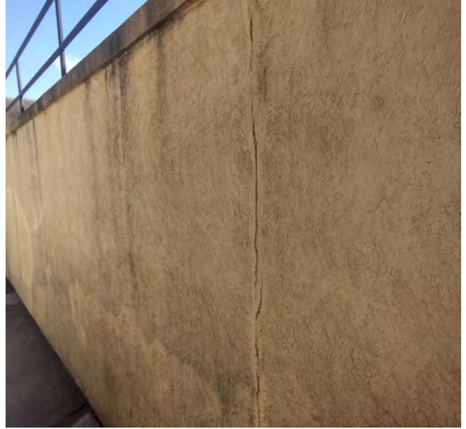
Bad or missing sealant, cracks, stained lamina.
