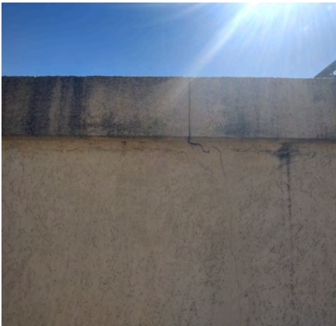
Large cracks and extensive lamina discoloration.
