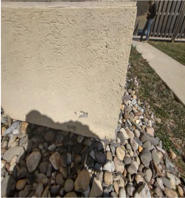
Missing sealant, impact damage and lamina discoloration.
