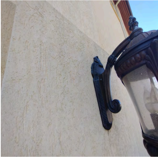
Bad or missing sealant throughout.
