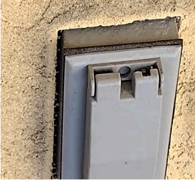
Bad or missing sealant, cracks, stained lamina.
