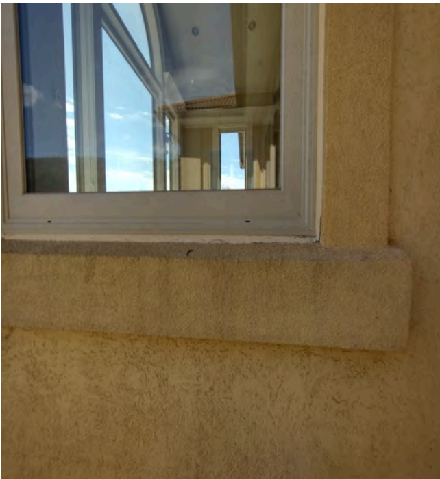
Missing sealant, impact damage and lamina discoloration.
