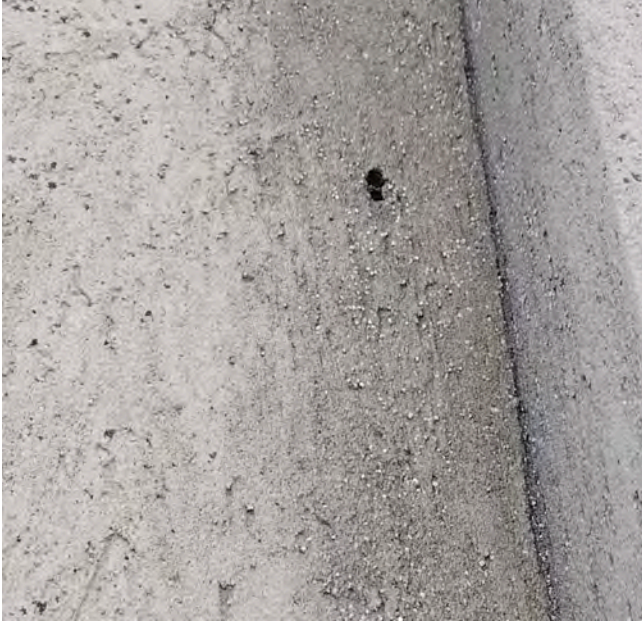
Impact damage and extensive erosion (no downspout)
