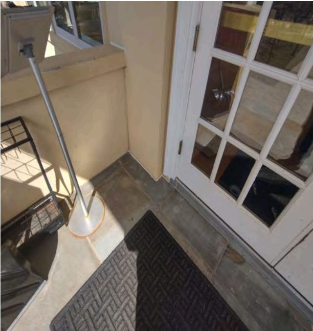
Missing sealant, impact damage and lamina discoloration.
