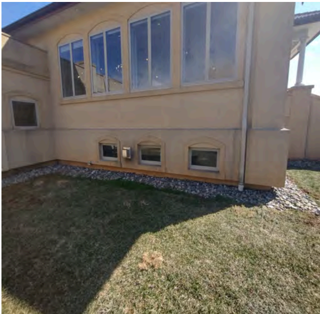
Impact damage, bad or missing sealant, cracks and stained facade.
