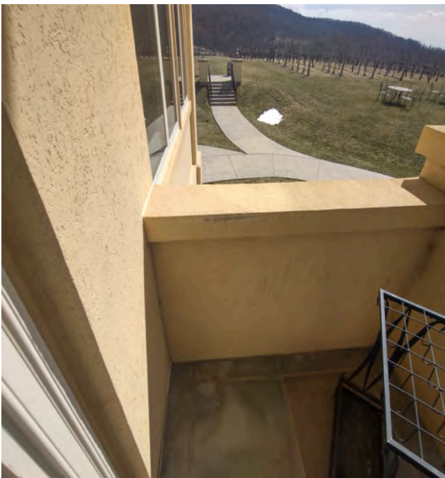
Missing sealant, impact damage and lamina discoloration.
