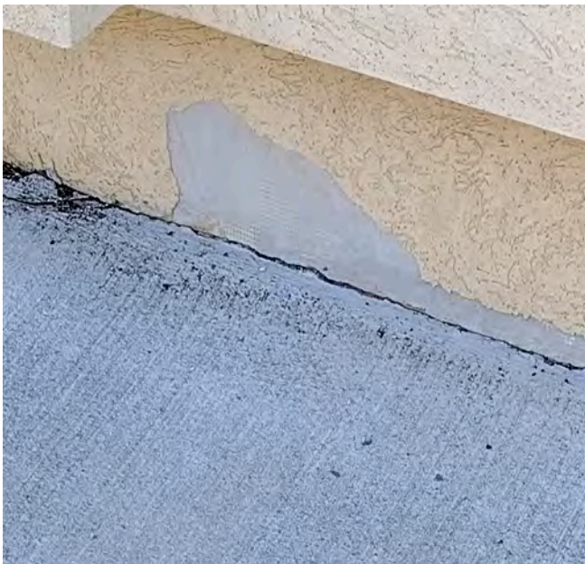
Lamina delamination.
