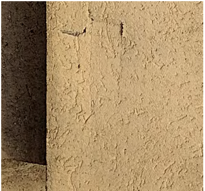
Impact damage & cracks throughout lower section of building.
