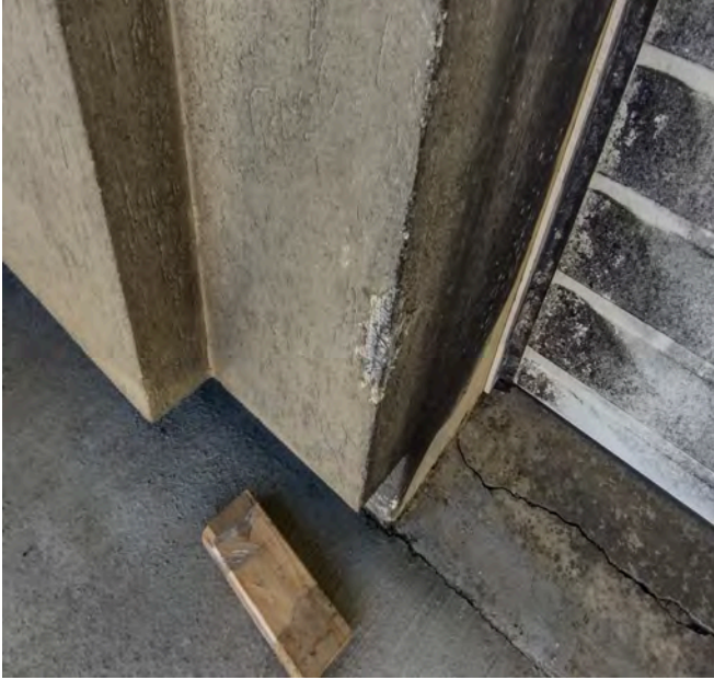
Impact damage, cracks, stained lamina.
