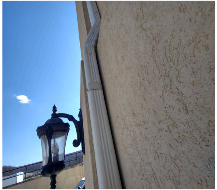
Bad or missing sealant throughout.
