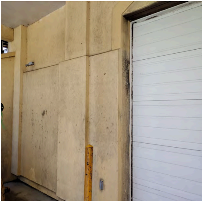
Impact damage & cracks throughout lower section of building.
