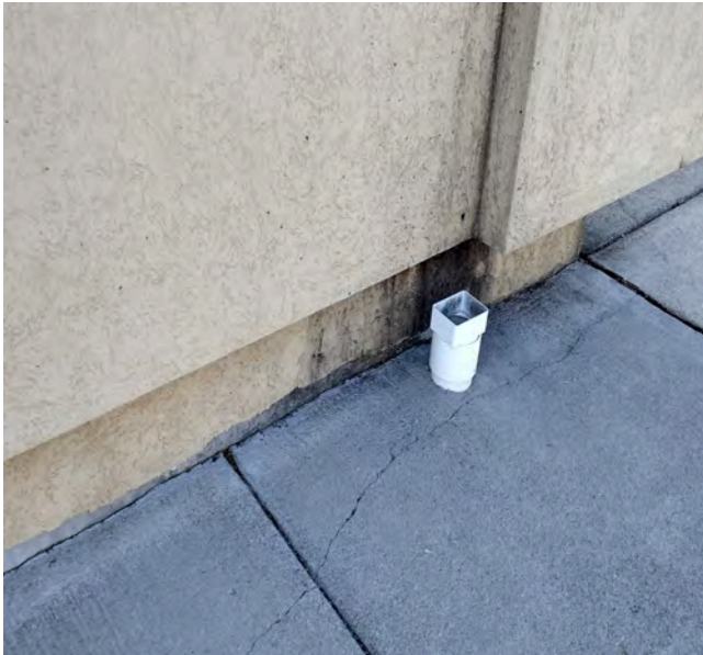
Damaged lamina and cracks.
