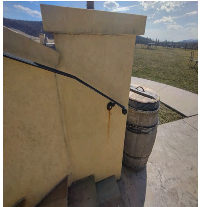
Missing sealant, impact damage and lamina discoloration.
