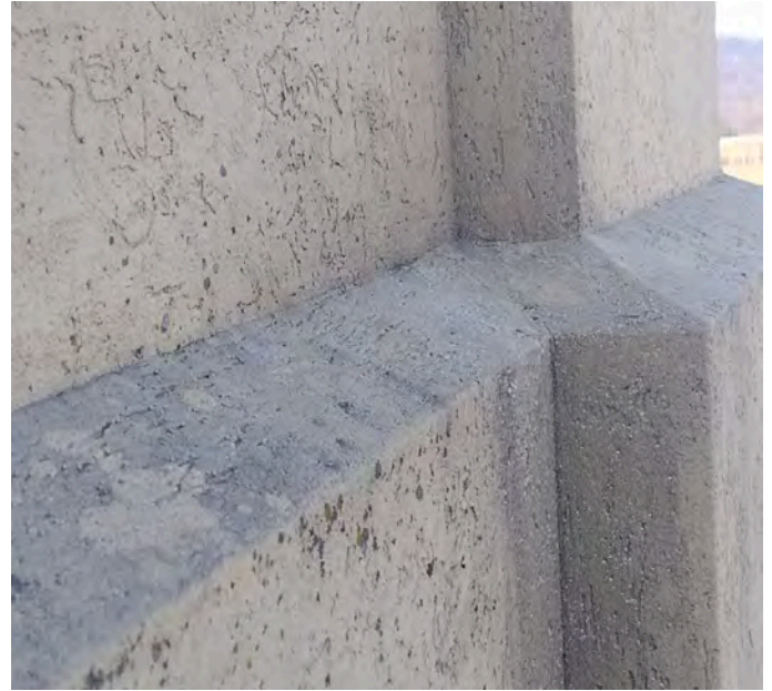
Impact damage and extensive erosion (no downspout)
