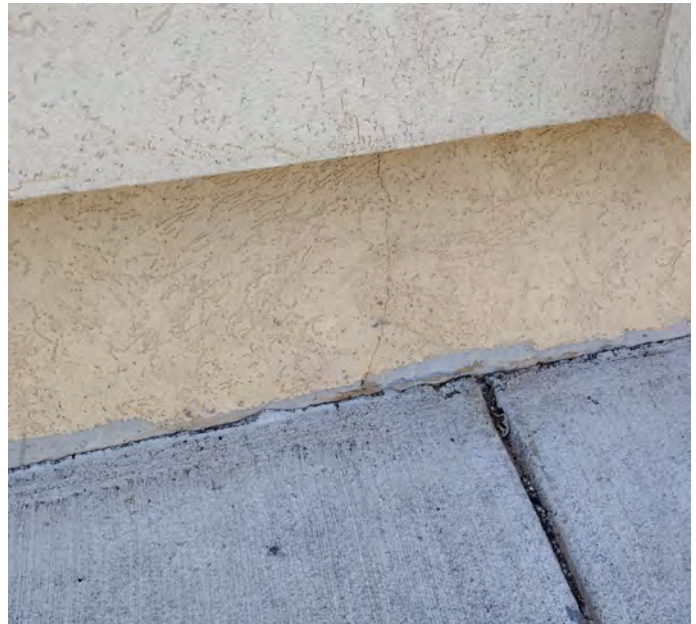
Cracks & delamination.
